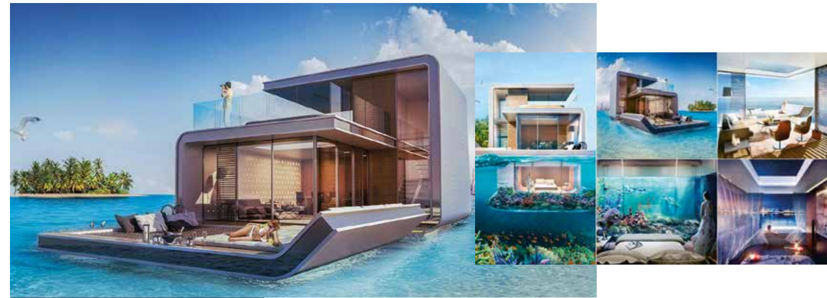
The Floating Seahorse villas (42 villas), Dubai, U.A.E.
